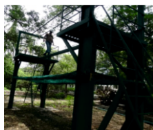
Height pass facility
